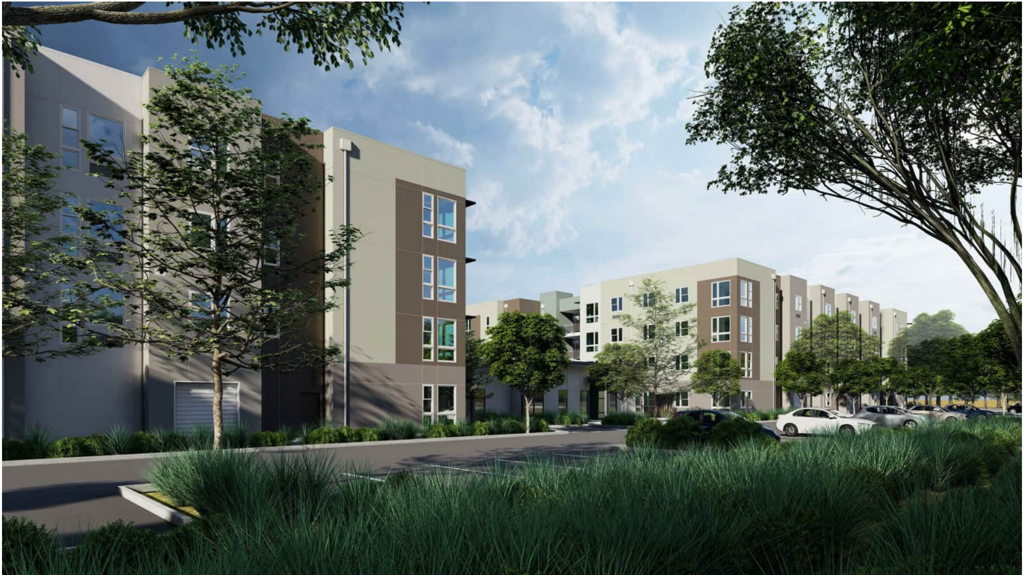
View from the North Property Line
